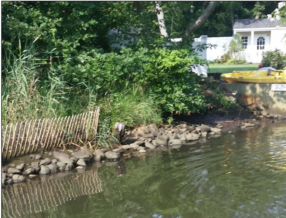
Portions of shoreline on residential properties have rock and debris reinforcement.
