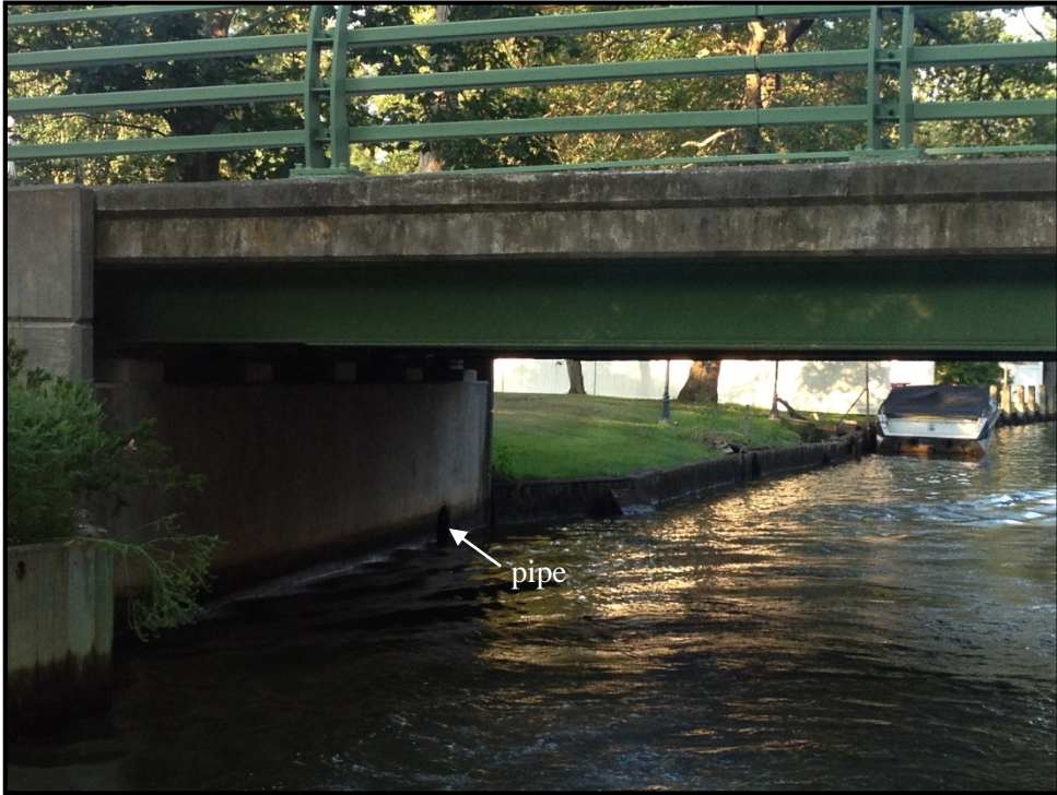
Stormwater outfall pipe from roadway is shown above
