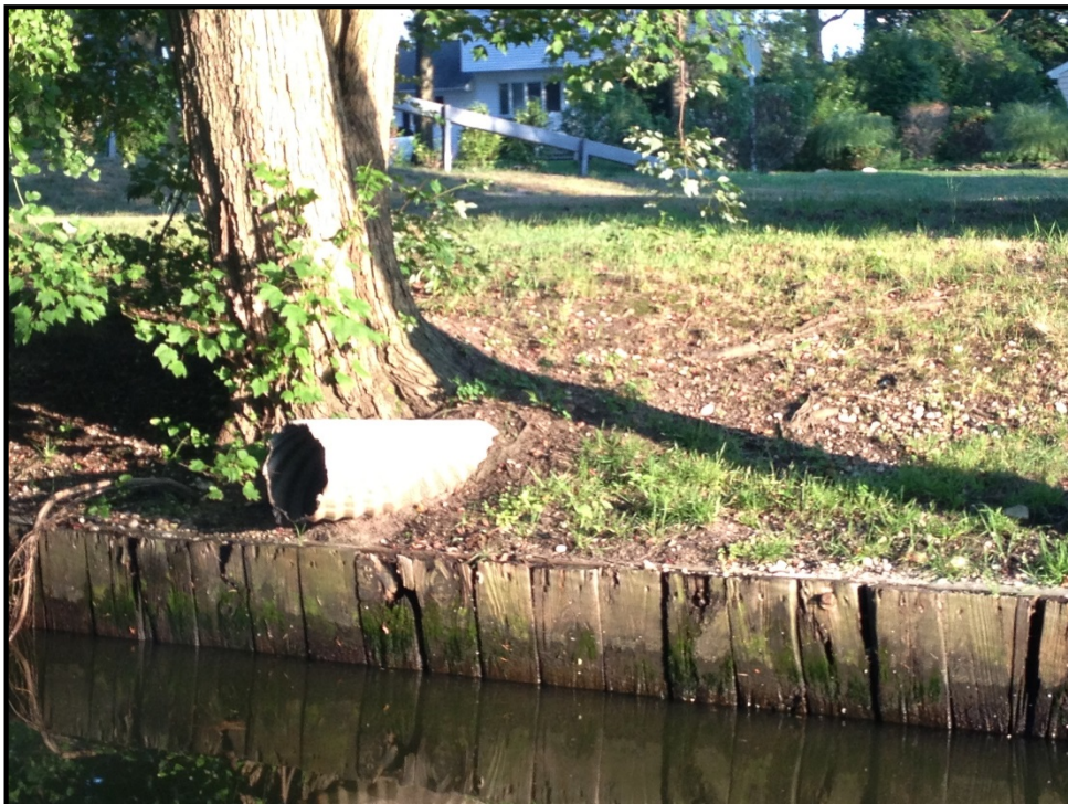
Stormwater discharge pipes of various sizes are located along canal.
