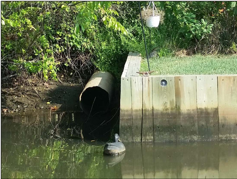
Stormwater outfall discharge to the canal.
