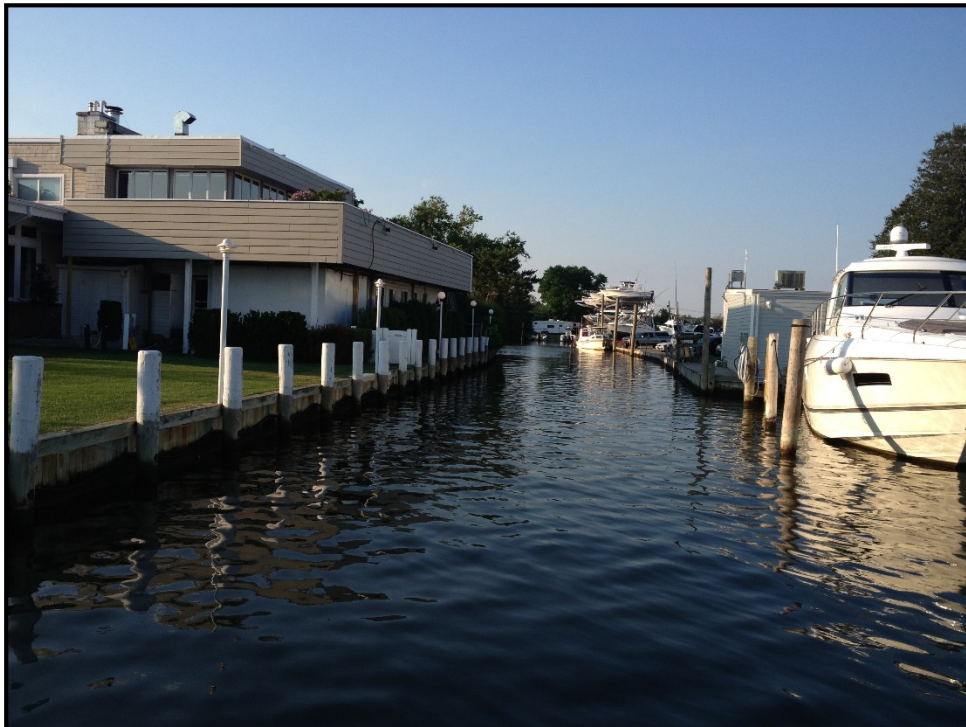
Buildings and homes are in close proximity to canal edge.
