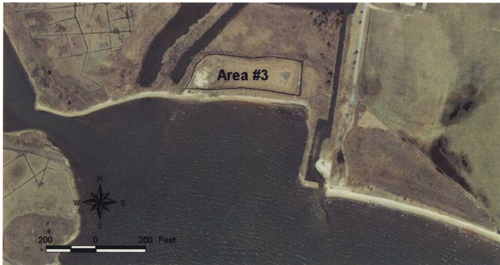
Area #3 Owner: St. John's University Approx. 1.3 ac. 15,000' pumping distance
