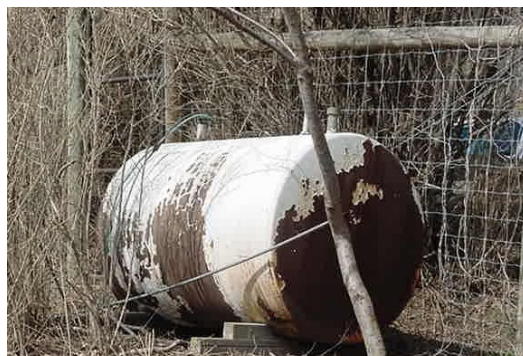
An old fuel tank that was eligible for funding.
