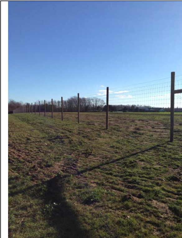
Best Management Practice—Deer Control Fence Standard 382A Woven Wire
