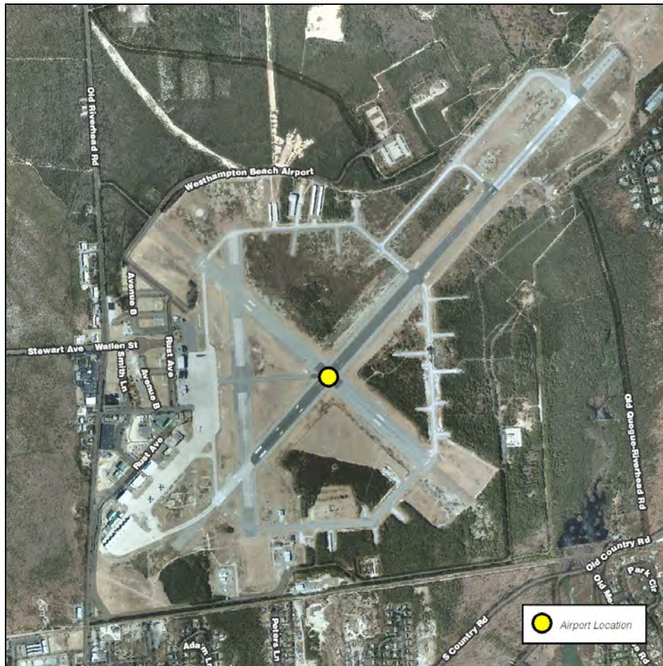
Figure A-55: Aerial View – Gabreski Airport
