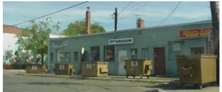
Figure 70 - Multiple dumpsters clearly visible from municipal parking lot off South Ocean Avenue.
