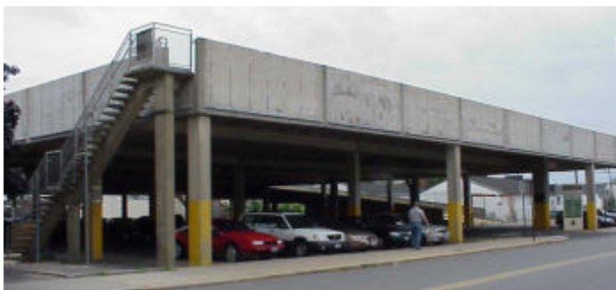
Figure 32 - Public parking and parking structure (lot #3) on the south side of Lake Street.
