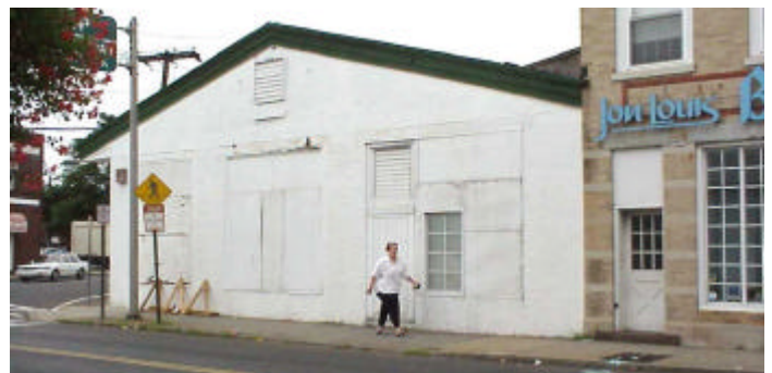
Figure 56 - Vacant Swezey's building on the southeast corner of North Ocean Avenue and Oak Street.
