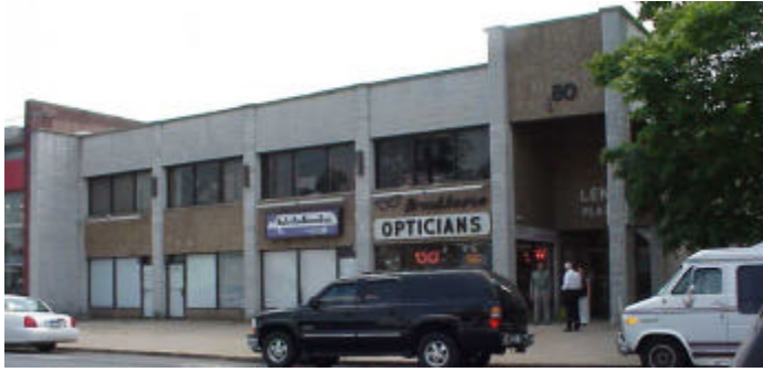
Figure 86 - Windows of occupied storefronts that are walled up, darkly tinted, or closed off with blinds or shades are uninviting to pedestrians, shoppers, and visitors.
