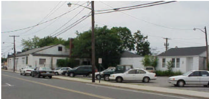
Figure 77 - Vacant bowling alley parcel on the west side of Havens Avenue, looking south. This narrow parcel would contain the new Havens Avenue if the streets were aligned.
