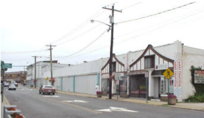
Figure 21 - Vacant stores on the west side of North Ocean Avenue north of Main Street.
