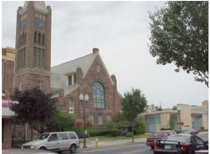
Figure 15 - Institutional and office uses are prevalent in downtown Patchogue.
