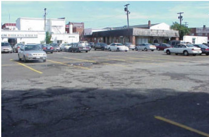
Figure 62 - Poorly paved municipal parking lot (#6) in downtown Patchogue.
