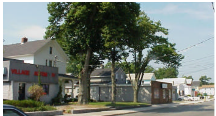
Figure 45 - Former homes on the south side of Terry Street partially converted to commercial uses.
