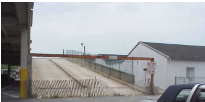
Figure 33 - Ramp to second level of parking structure, currently inaccessible.
