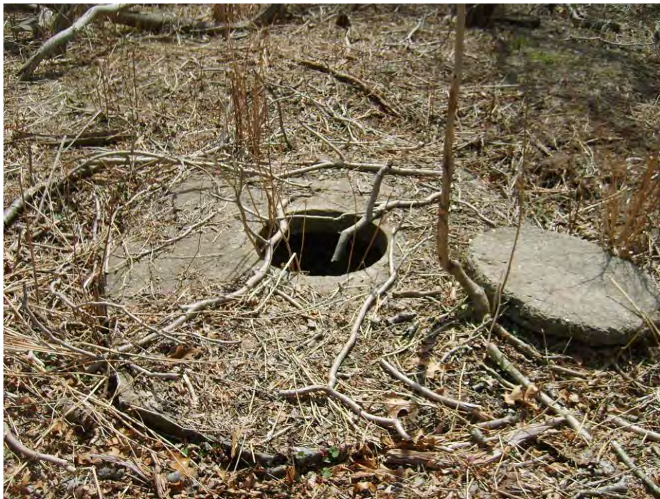
View of one of the two identified leaching pools located east of the former hangar. The other structure was of similar construction.
