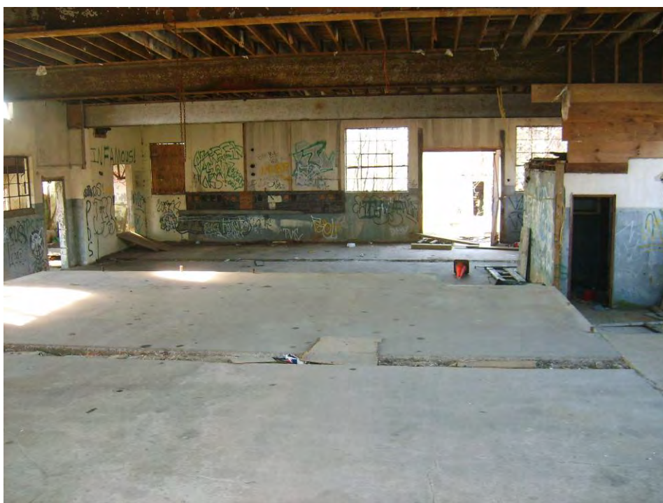
Interior view of northern farm building showing trench drains which appear to have discharged to the east.
