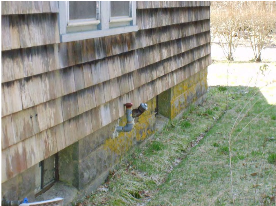
View of fuel oil tank fill and vent, typical of each of the three homes.
