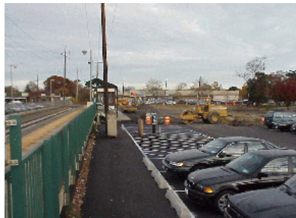
Figure 21 - Islip railroad station parking lot undergoing reconstruction in 1999.
