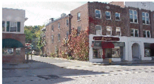
Figure 20 - Small-scale multi-unit housing constructed above storefronts adds to the economic vitality of a downtown area.
