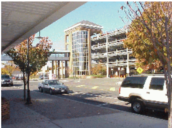
Figure 2 - Parking garage built at the Ronkonkoma train station in the 1990s.
