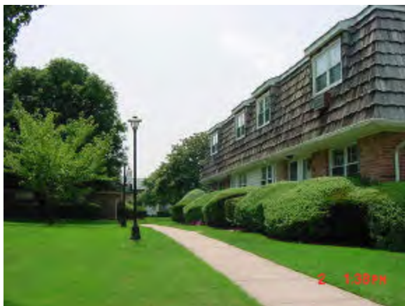
Figure 12 - Birchwood on the Green Co-ops in Oakdale, about one-half mile from the Oakdale station.
