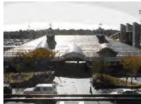
Photos above show the reconstructed LIRR Ronkonkoma Train Station with surrounding mixed uses.
