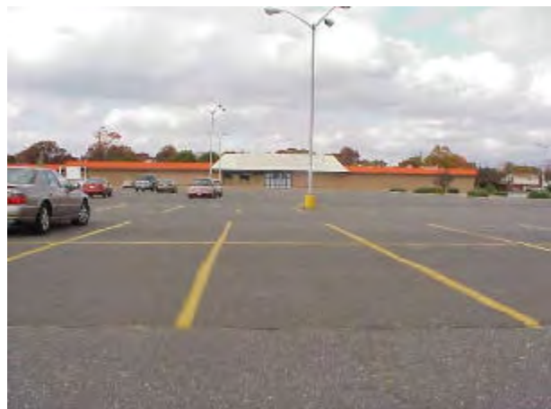
An abandoned part of a shopping center in Babylon Town
