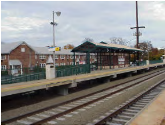
Pictured is a garden apartment complex adjacent to and existing rail road station.
