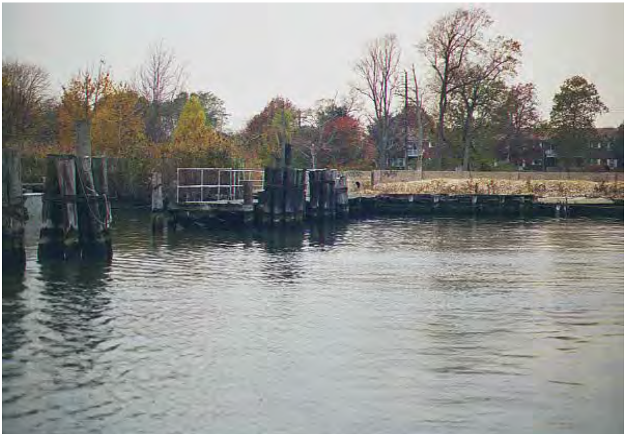
Photograph 4 - Former oil terminal property owned by Amerada Hess Corporation in the Southwest River Segment.
