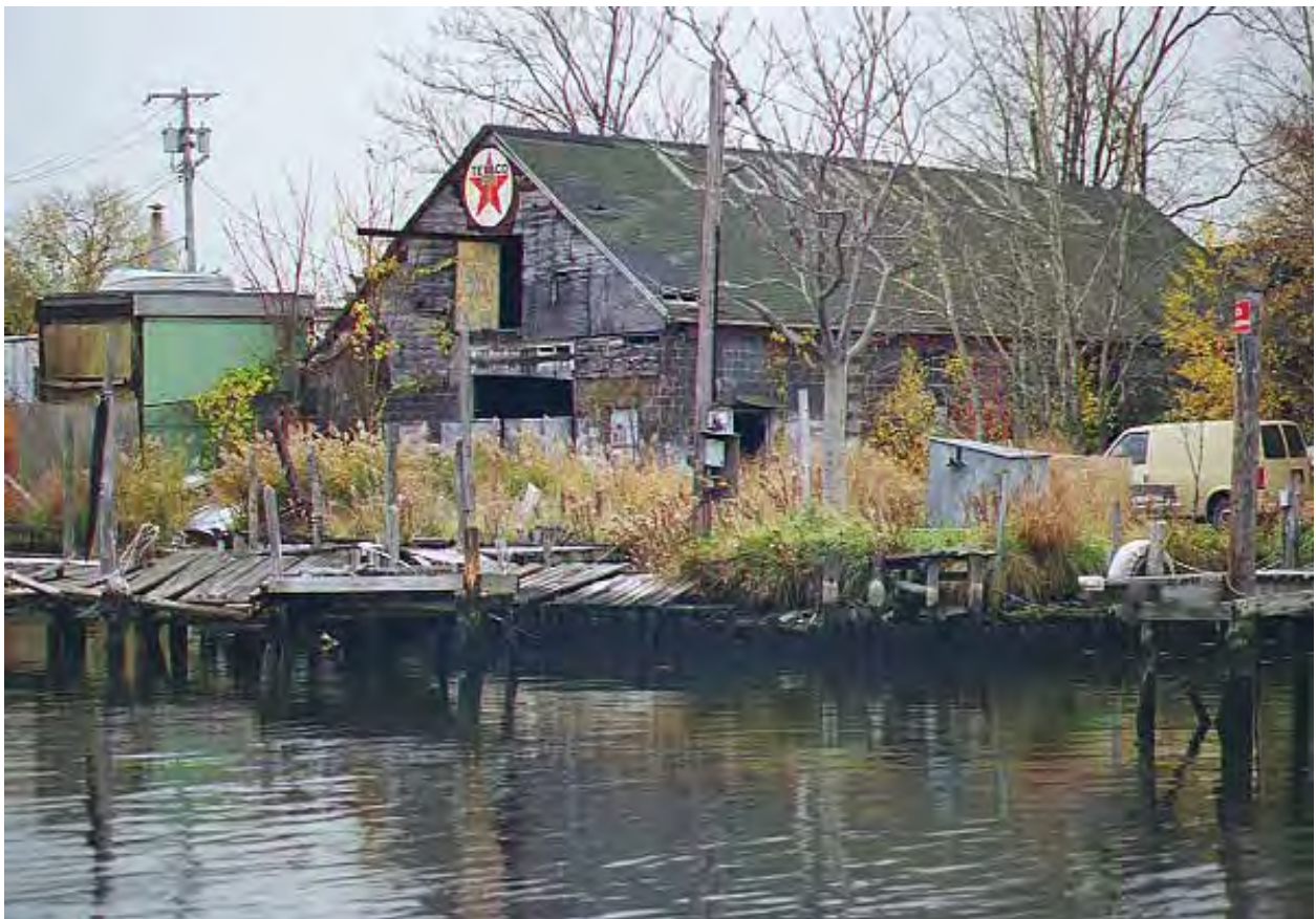
Photograph 5 - Deteriorated Connelly boatyard facility on site having water-related development potential.
