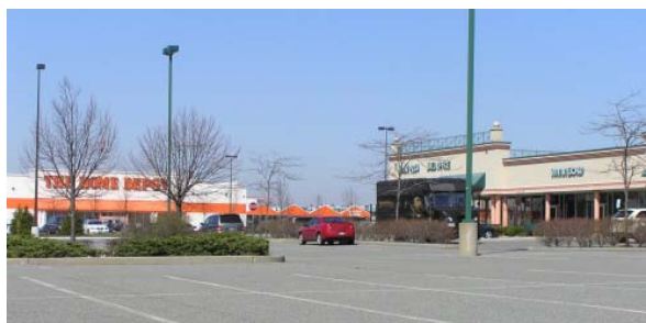
Bellport Outlet Stores and new Home Depot North Bellport, April 2008.
