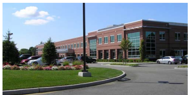
New office building on Hospital Road in East Patchogue.
