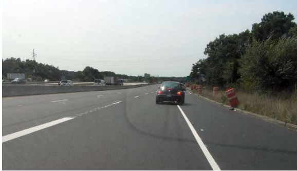
The Sunrise Highway North Service Road at Beacon Drive, near the exit ramp off Nicolls Road.
