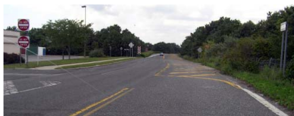
Two-way service road and awkward entrance to the Bellport Outlet Center.
