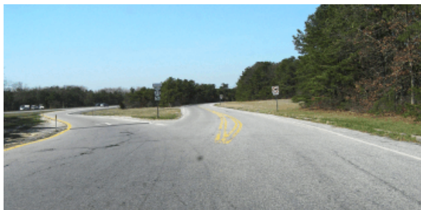
Confusing two-way service road and Sunrise Highway entrance ramp in East Patchogue.
