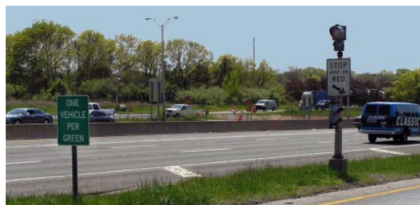
Ramp metering on the Long Island Expressway.
