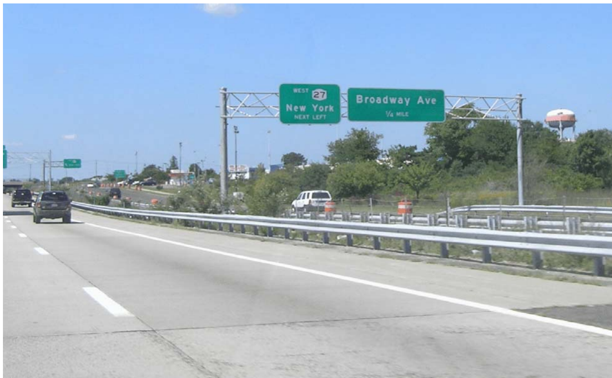
Sunrise Highway in Holbrook after completion of limited access construction, with three travel lanes and two service road lanes in each direction.
