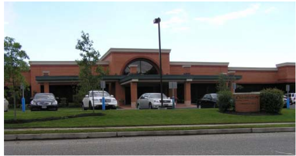
New light industrial and office uses, such as this new building in the North Bellport/ Yaphank area are encouraged.
