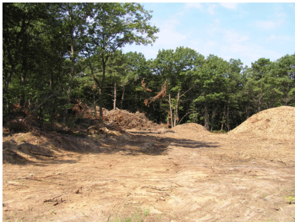
New residential subdivision beginning construction in East Patchogue.
