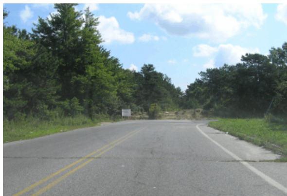
End of the two-way Sunrise Highway south service road in North Bellport.
